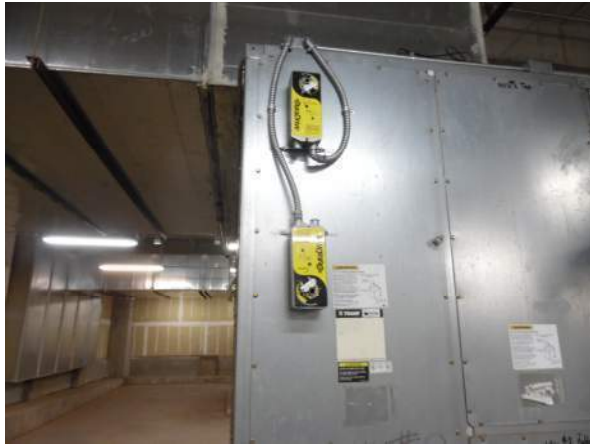
Photo #7 Typical split return air actuator below with outside damper actuator above
