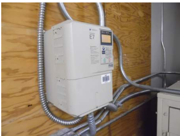
Photo #11 VFD serving AHU 3M1.
