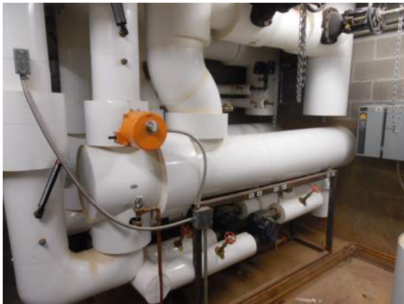
Photo #9 The steam heat exchanger converts steam to hot water for heating water service in the College of Medicine Building.
