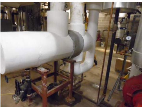
Photo #11 Steam bundle heat exchanger serves three buildings from the basement mechanical room in the Atrium.
