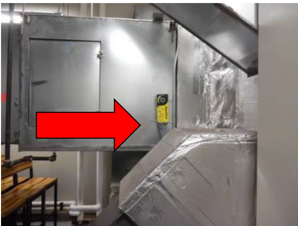
Photo #5 Typical relief fan with damper actuator for each floor necessary to achieve static air pressure design conditions when AHUs are in air economizer mode.
