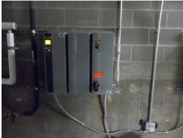
Photo #7 Two separate VFD's and disconnects serve CHW Pumps #1 and #2.
