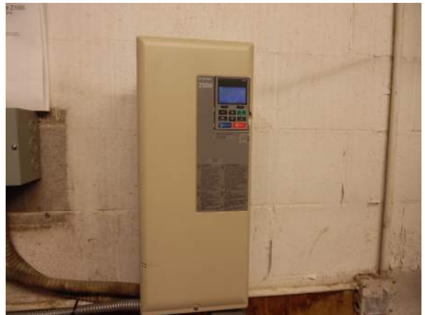
Photo #6 Typical variable speed drive (VFD) serves the chilled water pumps.
