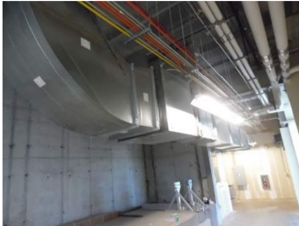
Photo #13 Exhaust fan for general building exhaust.
