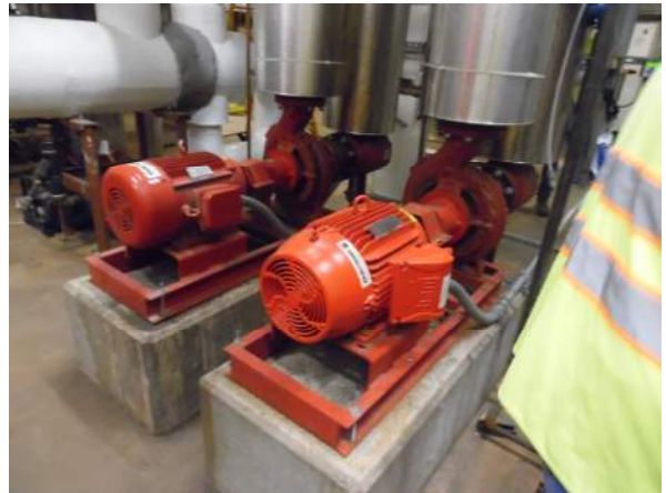
Photo #10 Lead/Lag hot water pumps which serve the Atrium and SAMIS buildings.
