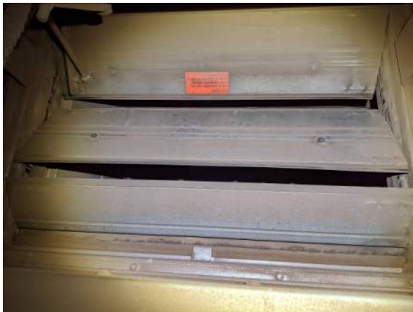
Photo #9 Typical condition of corroded and debris laden outside air dampers with airflow monitoring station.
