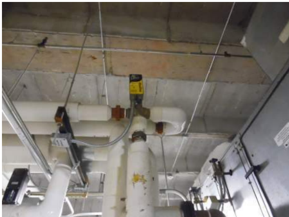
Photo #9 Typical 3-way hot water valve.
