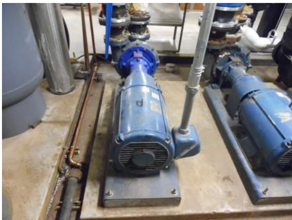
Photo #11 Dual chilled water pumps.
