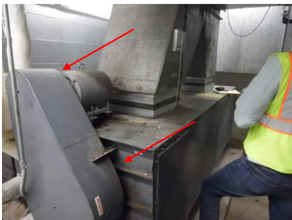
Photo #17 AHU 5N1 is a TRANE unit manufactured in 1979 that has noisy fan bearings.
