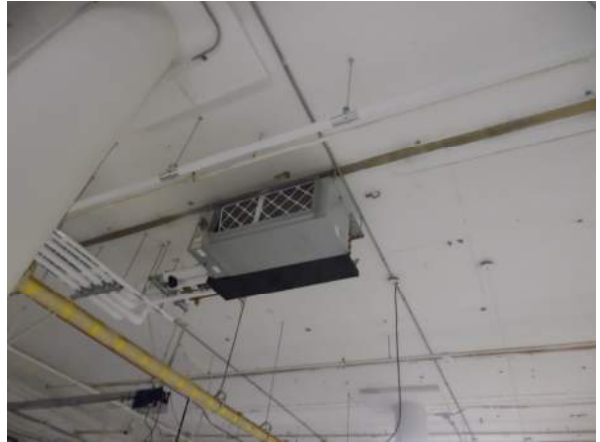
Photo #2 FCU serving the first floor four pipe system. This floor is being used for storage during an on-going renovation.
