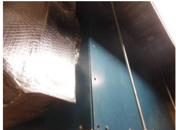
Photo #4 SF-1 and SF-3 serve the basement and first floor and assist to regulate building pressure.
