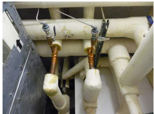
Photo #6 Hot water differential pressure sensors for the building are installed on the second floor.
