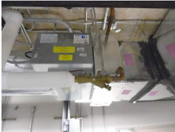
Photo #7 Typical Titus VAV box with reheat coil throughout the building.
