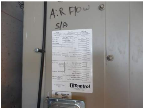
Photo #15 AHU-2 Gear Tag. M# ITF-DHRE-135 S# T016772-002-00 and is a Tentrol brand unit also features 12 supply and 12 return fan arrays.
