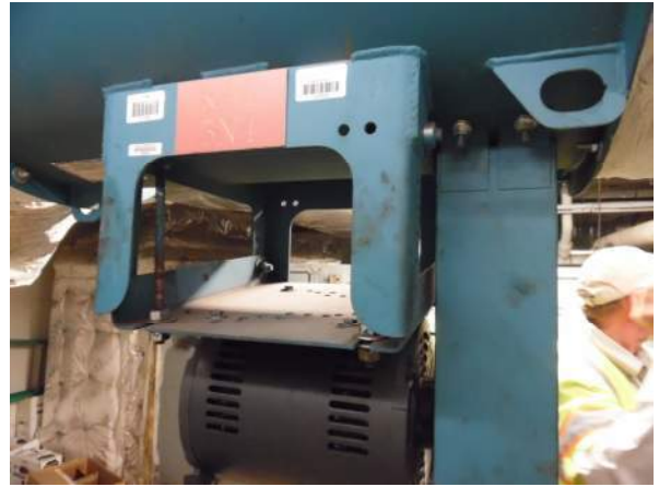
Photo #14 Separate supply and return air fans are used for AHU 3N4 on the third floor.
