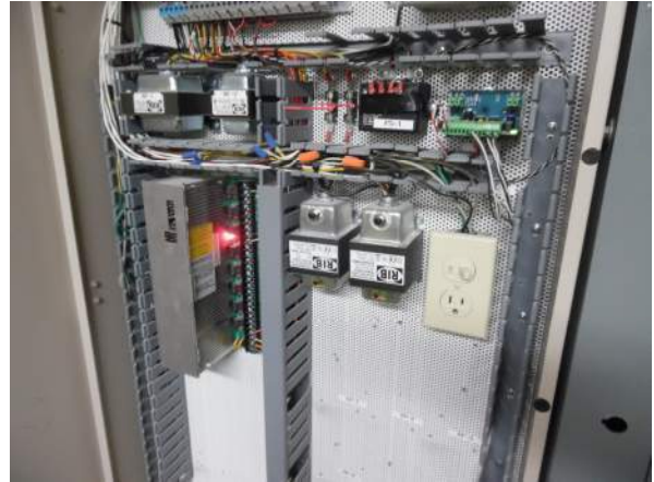
Photo #2 Automated Logic Controls (ALC) controllers have been upgraded since building was originally constructed.
