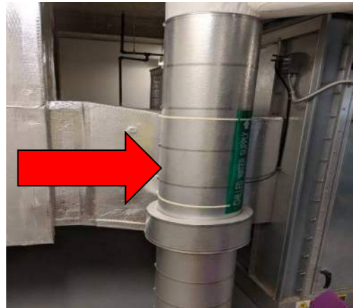
Photo #8 Access to clean and maintain sensor for outside air flow monitoring station is obstructed by chilled water piping in mechanical room.
