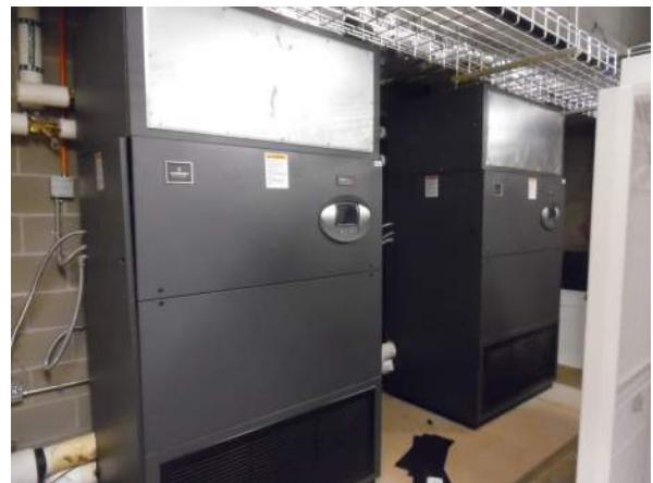
Photo #12 Dual Liebert Units are installed and serve the basement area of the College of Medicine Building.
