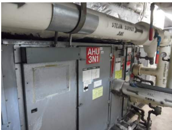
Photo #11 AHU 3N1 has been abandoned and is not in service.
