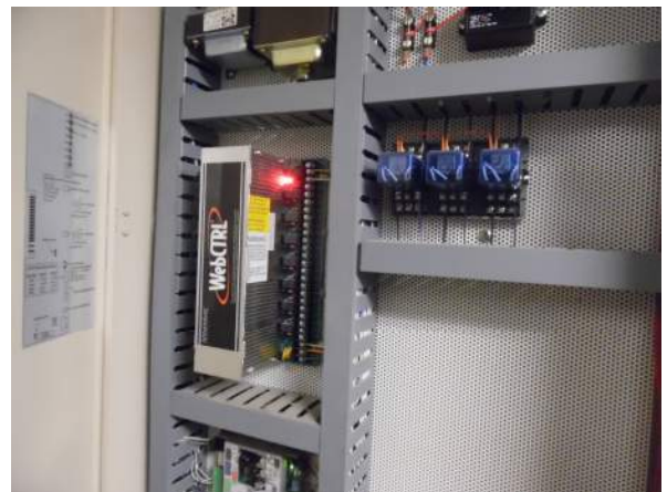
Photo #6 Typical ALC type enclosure with relays, transformers, and BAS controllers.
