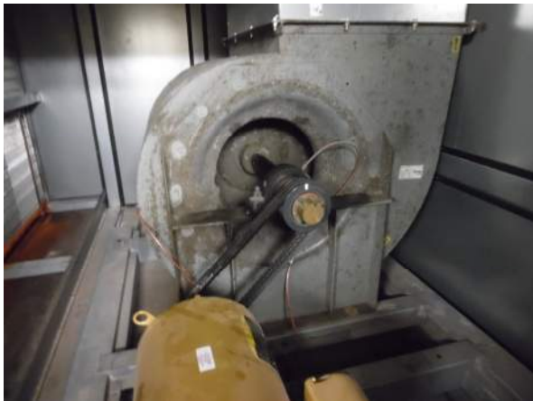
Photo #15 AHU 4N1 is a McQuay unit manufactured in 2011 with a dirty blower section and dirty coils.
