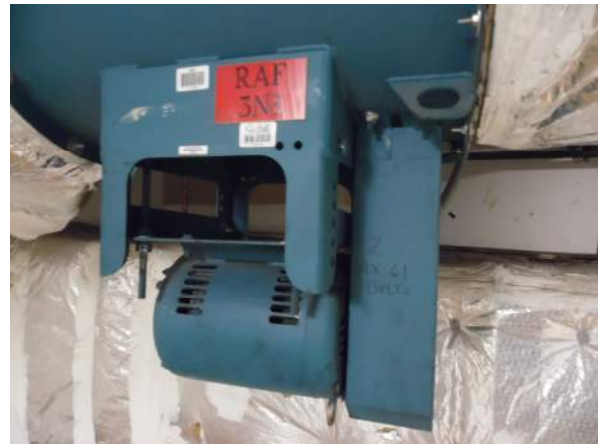
Photo #10 Separate supply and return air fans are used for AHU 3N3 on the third floor.
