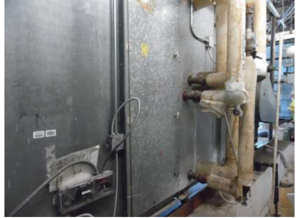
Photo #20 AHU 6N3 is a York unit manufactured in 1978 with outdated controllers.
