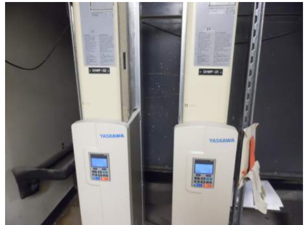
Photo #4 VFD's controlling chilled water pump #1 and #2.
