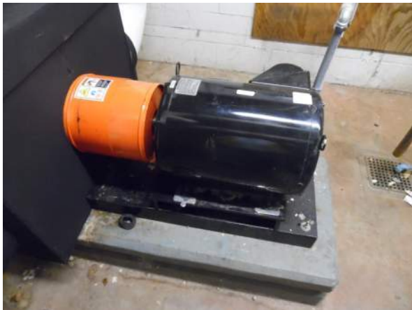
Photo #5 Chilled Water Distribution Pump #1.
