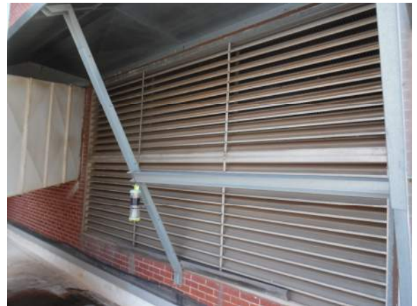
Photo #16 O/A damper array on the 7 th floor.
