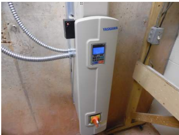
Photo #5 Two Yaskawa VFD's serve -SF#1 and SF #3 located in the basement mechanical room.
