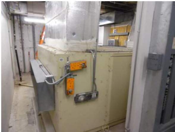
Photo #9 AHU 3M1 is a Temtrol unit serving the third floor.
