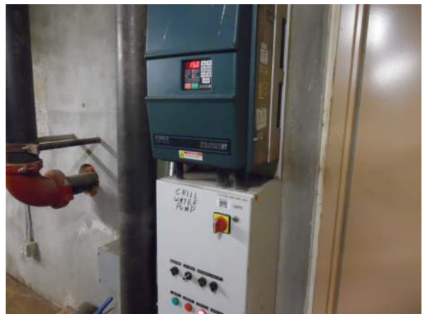
Photo #12 Defective chilled water VFD
