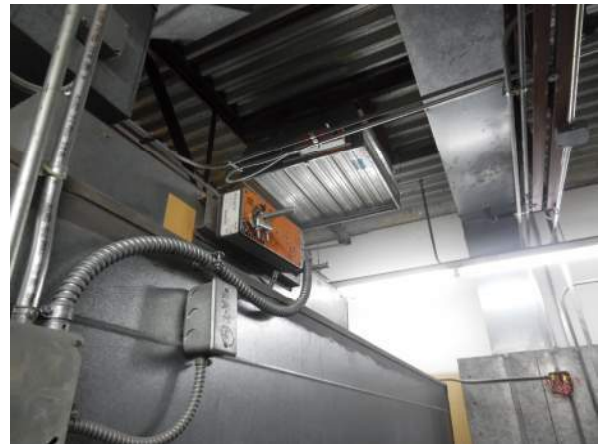
Photo #16 Relief air damper and actuator for AHU ventilation requirements.
