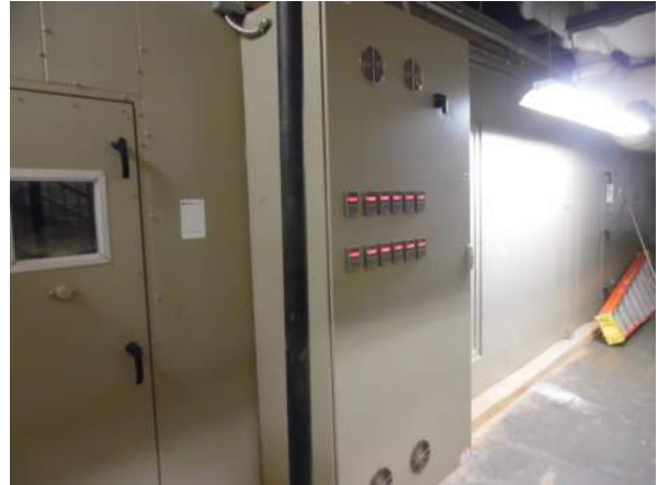
Photo #2 AHU-1 is a Temtrol unit in the basement and features 12 return air and 12 supply air fan arrays.
