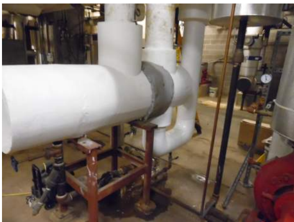
Photo #11 Steam bundle heat exchanger serves two buildings from the basement mechanical room in the OU Childrens Physician's building.
