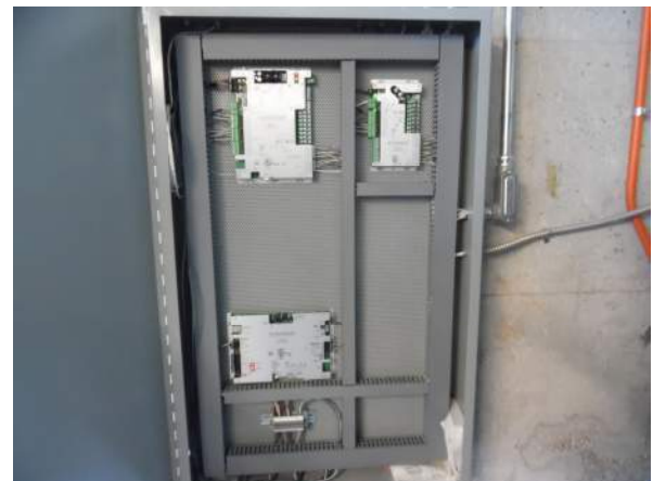
Photo #16 The Automated Logic controls were viewed by Terracon.
