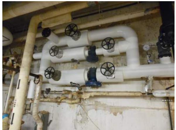
Photo #4 New steam piping, valves and usage meters were being installed at the Nicholson Tower.
