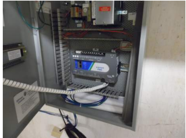
Photo #8 OUHSC Steam and Chilled Water Plant controller for collecting data related to utility metering.
