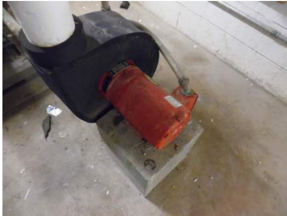
Photo #7 Fifth floor booster pump is served by a typical VFD.
