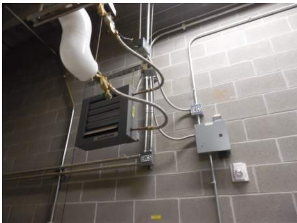
Photo #11 Unit heater serving basement mechanical area.
