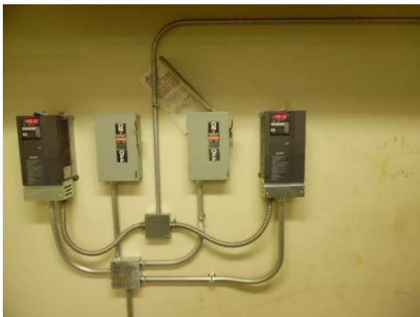
Photo #5 VFDs with electrical disconnects are utilized for flow control of the heating hot water distribution.
