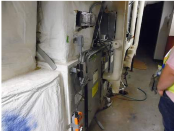
Photo #7 AHU 1M1 is a VAV multizone unit located in Rm# 1005 first floor.
