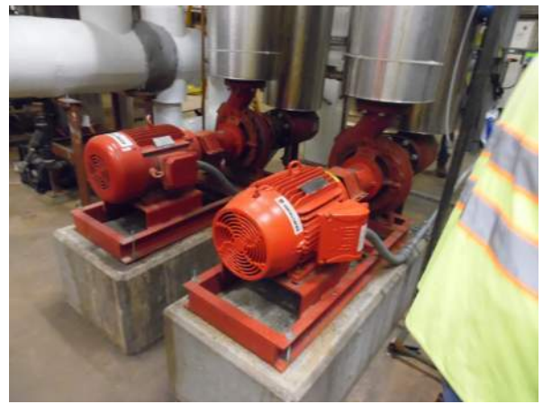
Photo #10 Lead/Lag hot water pumps which serve the Atrium and SAMIS.
