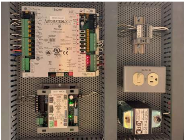
Photo #9 Typical ALC controllers for AHU -H5.
