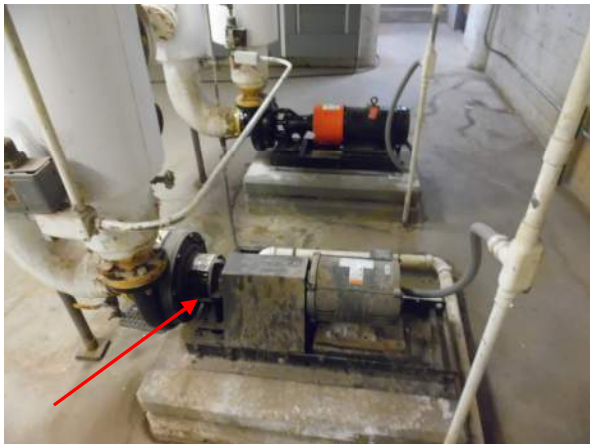
Photo #3 Heating Hot Water Distribution Pump #2 has noisy bearings and should be repaired.
