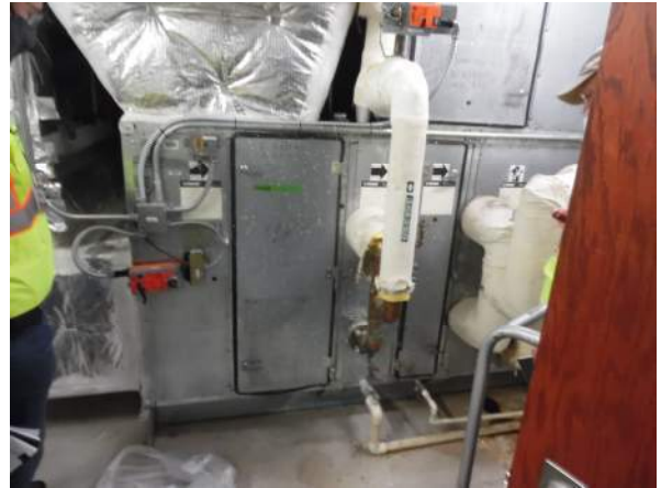
Photo #8 TRANE AHU 2M1 is a 1994 air handling unit serving the second floor of the OTC. S# K94J67844.
