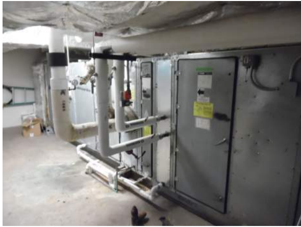
Photo #13 AHU 3N4 is a TRANE unit manufactured in 1994 that appears to have had the steam coils replaced by hot water coils.
