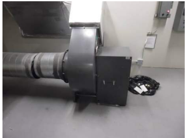
Photo #4 Typical constant volume exhaust fan serving each floor needed to achieve static air pressure design conditions.
