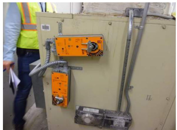
Photo #12 AHU 3M1 has return air damper control along with outside air control dampers and actuators.
