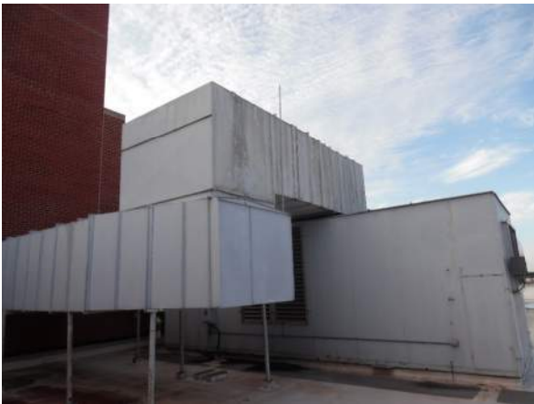
Photo #15 ERU abandoned on the 7 th floor roof.
