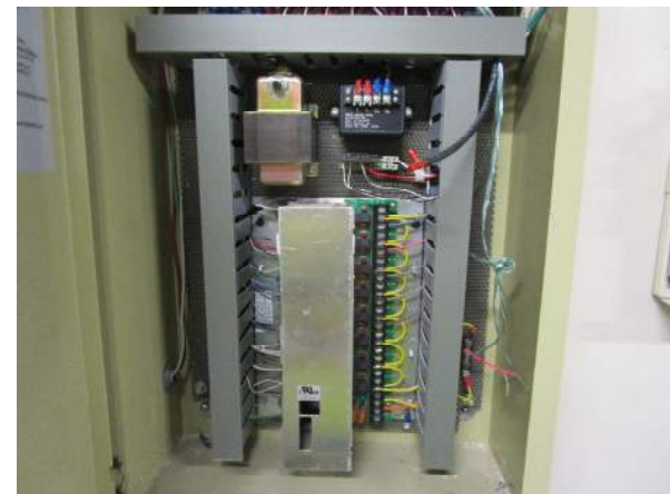
Photo #18 Retrofitted ALC controller for RFs and EFs.
