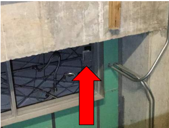
Photo #15 CO2 sensors are in the return air duct at each floor entering the chase.
