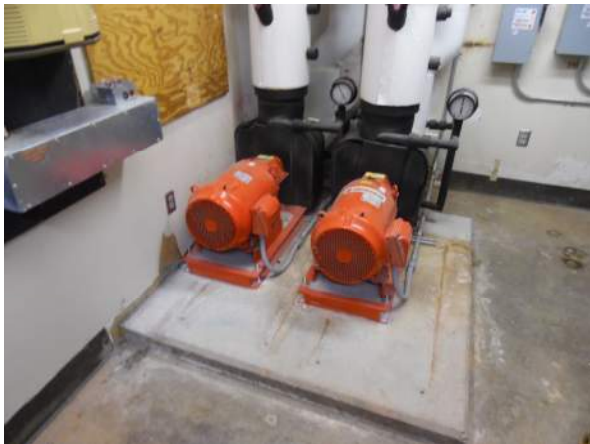
Photo #3 Lead/lag chilled water pumps serve the OTC building.
