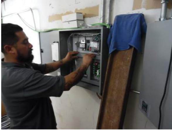
Photo #19 HVAC controllers for AHU 6N1 and the AAON FCU, serving the Auditorium were being updated.
