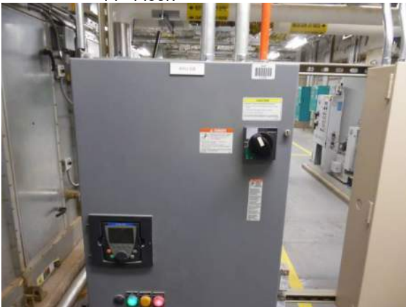
Photo #3 Typical AHU supply fan VFD controller that modulates fan speed.
