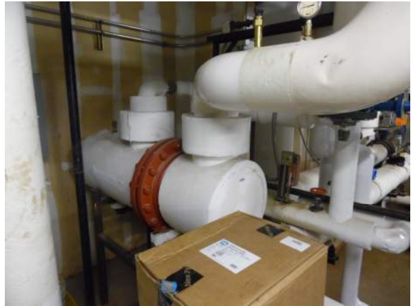
Photo #8 Heat exchanger for steam to hot water conversion.
