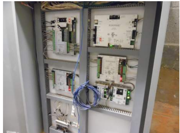
Photo #10 Terracon observed Automatic Logic Controls serving HVAC equipment in the College of Medicine Building.
