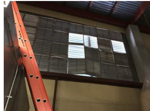
Photo #16 The gravity relief dampers need repair and or replacement.
