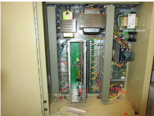
Photo #17 Typical retrofitted ALC controller for AHU.
