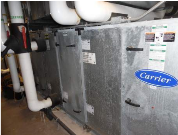
Photo #9 AHU 3 rd Floor Carrier
