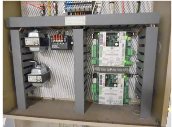
Photo #2 Typical ALC field controllers and panel that operates the exhaust and relief fans for each floor.
