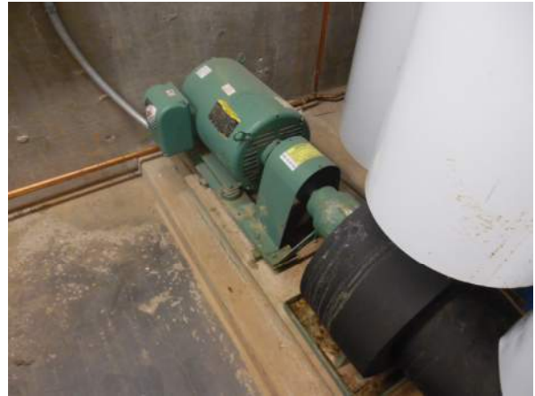
Photo #8 Dual Hot water pumps located in the basement mechanical room serve the College of Medicine Building.
