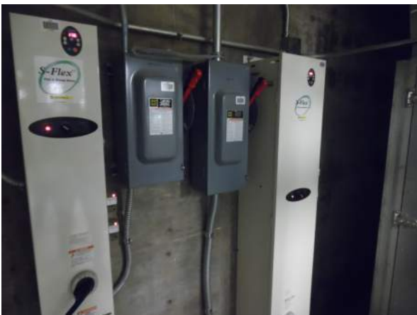
Photo #5 Typical electrical disconnects and VFD drives for serving AHU's.
