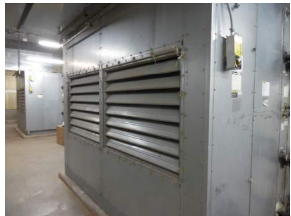
Photo #6 Typical return air damper with motorized damper control.
