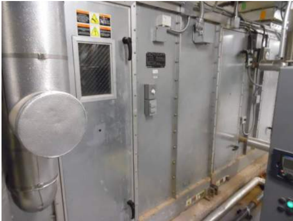
Photo #1 AHU F0 is a typical AHU serving the basement. Terracon viewed all air handling units on the basement through 14 th Floor.
