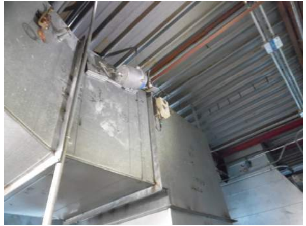
Photo #22 AHU 6N4 controls are outdated and partially operate on pneumatic air controls.
