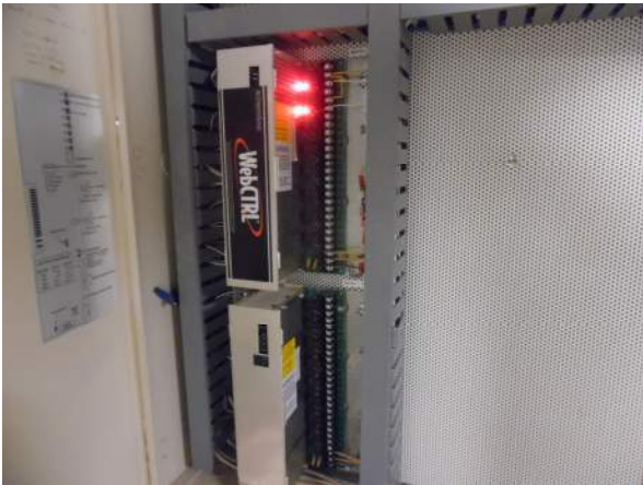
Photo #9 Typical ALC controllers for AHU -5G.
